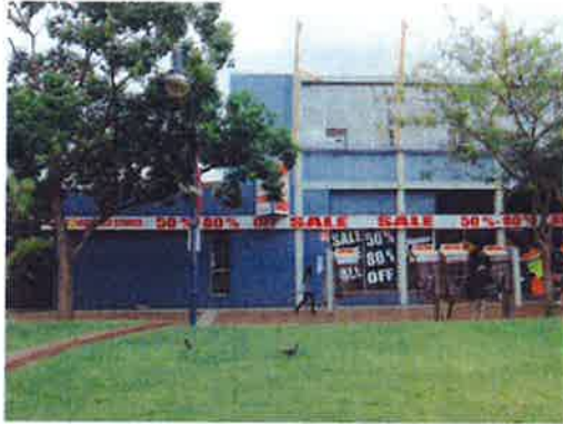
PICTURE 1 – VIEW OF BUILDING ON SITE FROM MACQUARIE STREET MALL
