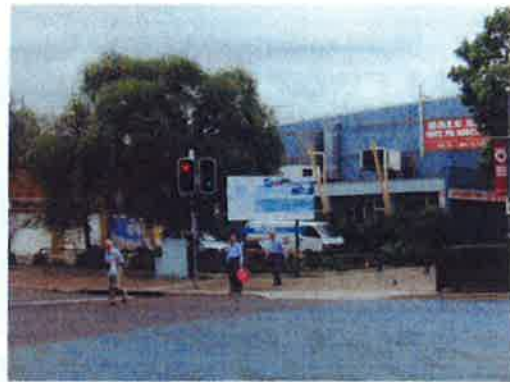
PICTURE 2 – VIEW OF CARPARK ON SITE FROM MOORE STREET
