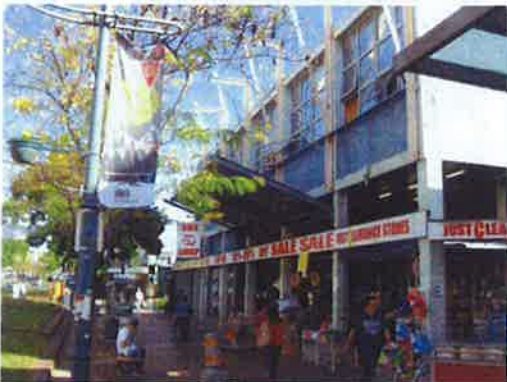
PICTURE 3 – MACQUARIE STREET FRONTAGE LOOKING SOUTH
